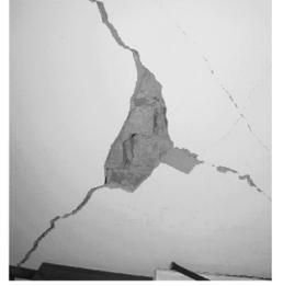
(b) 承重墙 X 形裂缝
