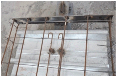
(a) 纵筋端部锚固措施
